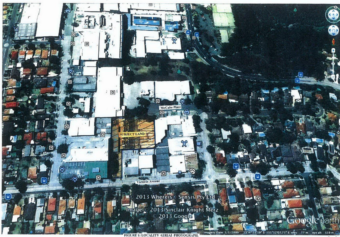
FIGURE 1: LOCALITY AERIAL PHOTOGRAPH.
